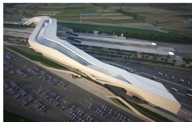
Napolit Afragola Station - Italy, 2017
